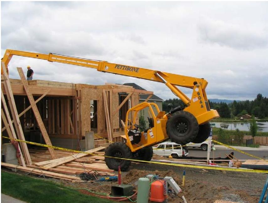
**Photo 1.** Forklift in position after the load came down. Note board pile in front of the forklift, preventing the forklift from getting closer to the second story.
