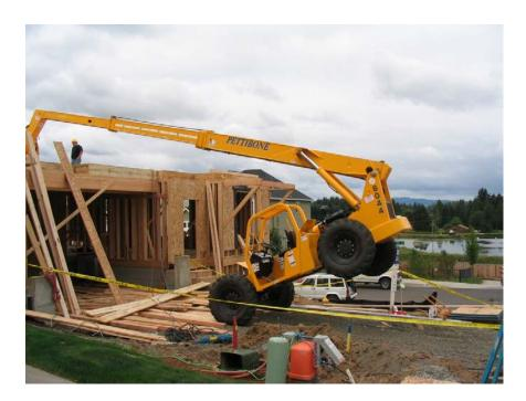
Photo 1. Forklift in position after the load came down. Note board pile in front of the forklift, preventing the forklift from getting closer to the second story.
