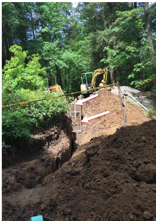
Figure 1. View from front of house: area of incident showing placement of shoring; collapse occurred in between the two pieces of shoring spaced 15 feet apart (indicated by arrows)
